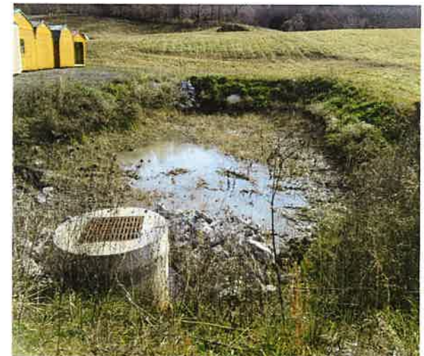
E&S Detention Pond
